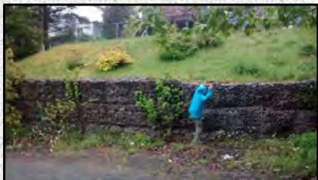
However, there is always an energy barrier to overcome...
