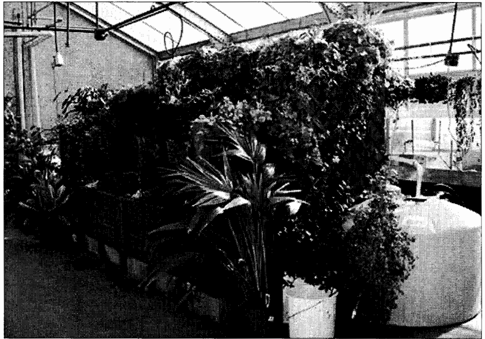
The breathing wall, filtering airborne contaminants through a wall of wet moss.
